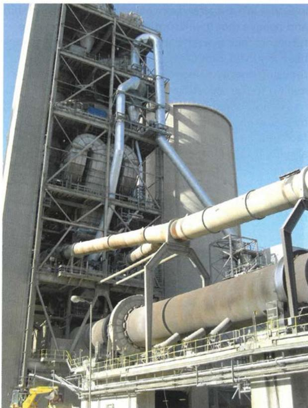
Kiln bypass at Ketton cement plant.
